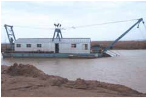
The dredge floats in the water-filled quarry as the cutting arm descends to the bottom.
